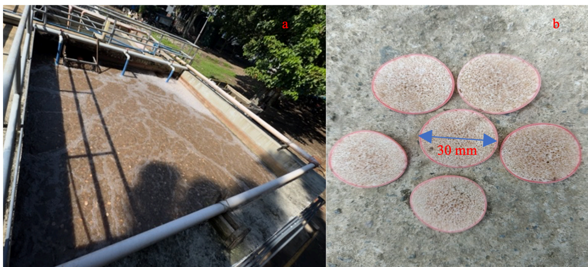
Fig. 2 a) MBBR Reactor, b) Biochips with attached biofilm.
